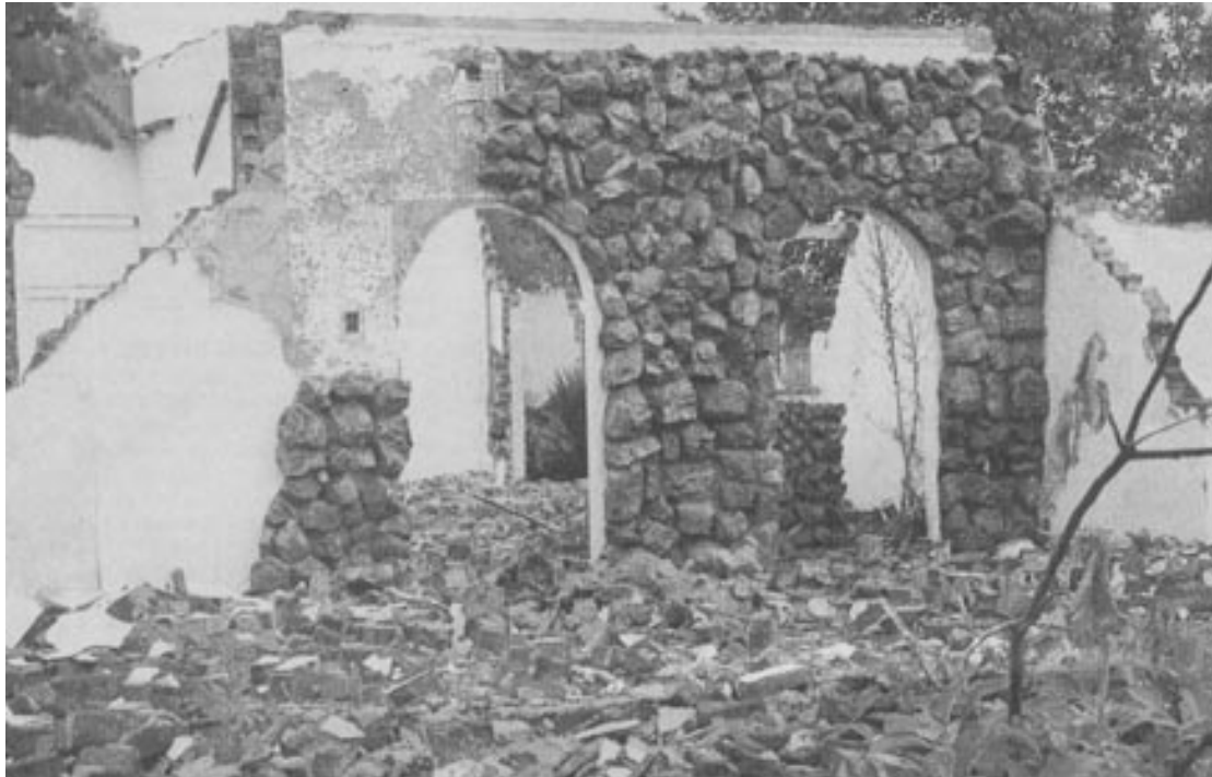
The remains of a house – literally dismantled brick by brick by squatters – in the Mapleton small agricultural holdings area on the East Rand. Similar scenes are to be found up and down the province.
